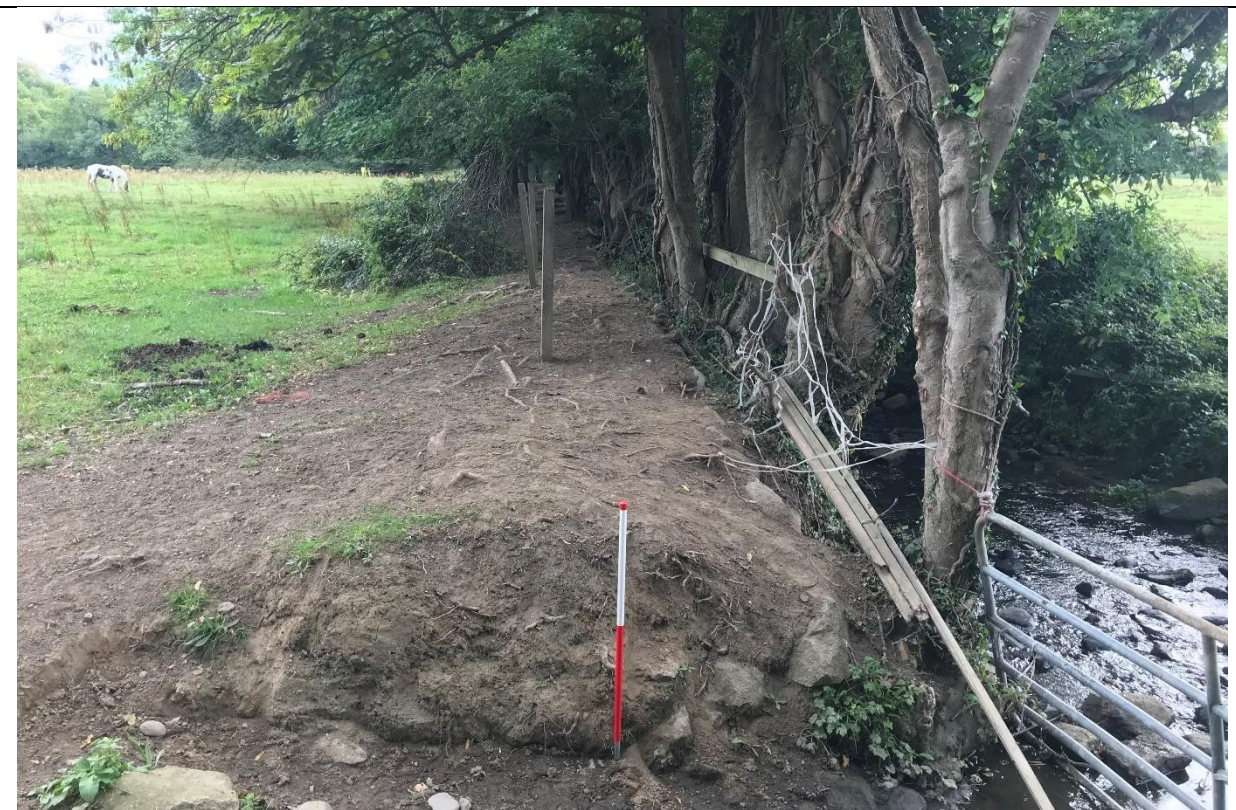
Plate 13.7 Earthen embankment along northern perimeter of stream, facing east
