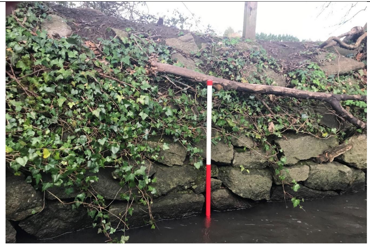
Plate 13.15 Example of stone facing on stream cutting, facing north
